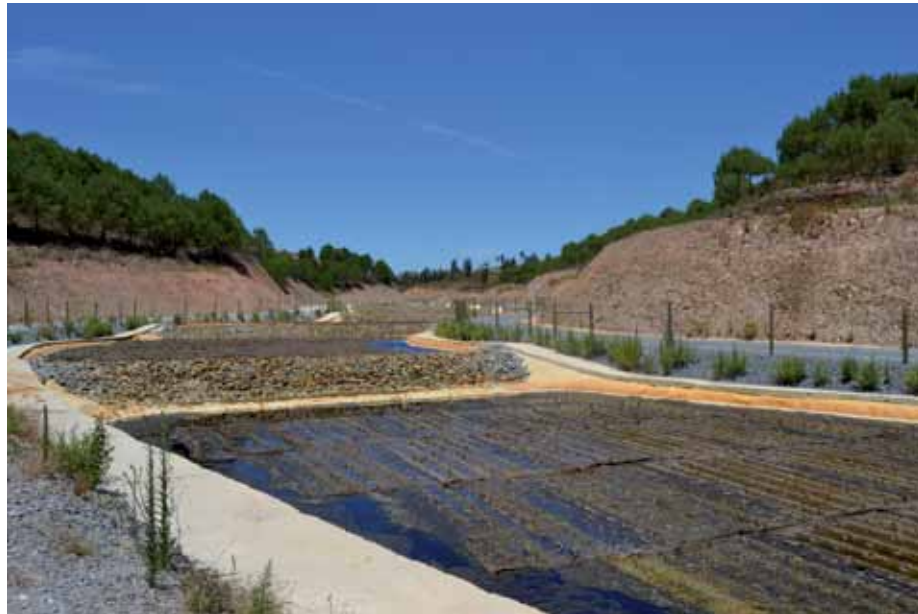
Figure 7. Partial perspective of the wetland system installed at Lousal
